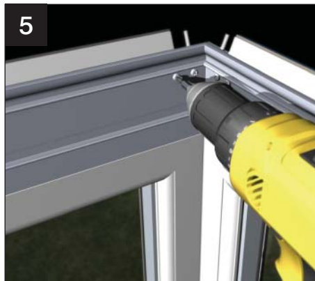
5 Securely fit the two M5 x 12mm tap screws.
