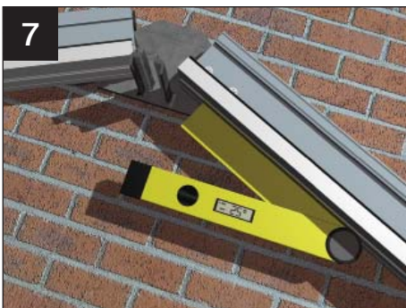
To set the height of the ridge, refer to the component location plan which states the height from the top of the frames to the underside of the ridge hanger. For added peace of mind use an "angle fix" check the starter bars are at the correct pitch. Chalk/pencil a line on to the wall to mark the pitch line.
