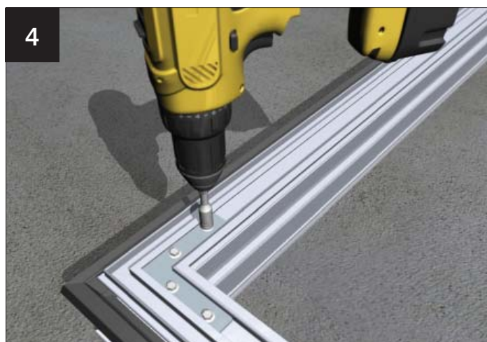
Fasten both fixings in both cleats on every corner
