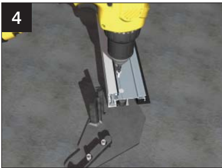
On the ground, away from the conservatory, offer up the first starter bar. Fasten using the set screws provided - do not over tighten.
