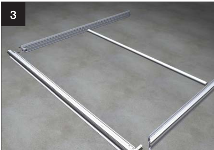
Layout the pieces of the lantern eaves beam.
