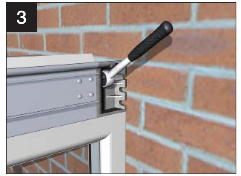
Where the eaves beam sits against the host masonry wall, it has a structural moulding attached to the eaves beam. This has three fixing positions cast into it to allow attachment into masonry – choose the hole that directly lines up with solid masonry and drill a 10mm hole into the host wall. Attach the structural moulding using the M8x80mm anchor supplied. Silicone seal the gap where the moulding attaches to the eaves beam.
