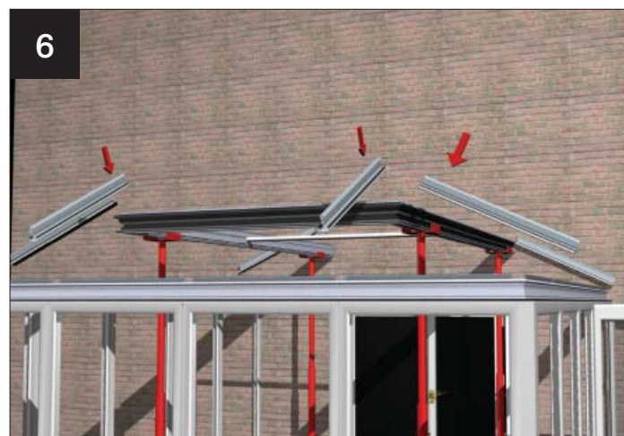
Now the Lantern eaves beam is assembled into a one piece structure, temporarily support it. Attach the glazing bars according to the component location plan. Tighten the bars, at the pagoda beam end first and then at the main eaves beam second.
